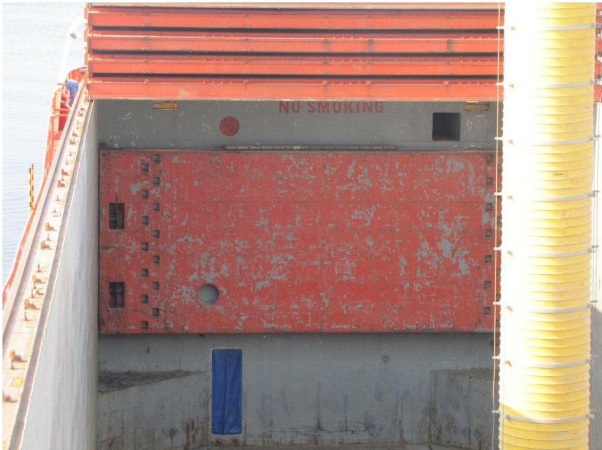
Bulkhead / tweendeck pontoon stored away.
